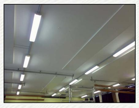
This installation method is generally utilised when there is insufficient ceiling void, or the void is inaccessible. Panels are supplied with colour matched end caps to close the ends of the runs. Mounting is achieved by first securing the supplied steel brackets to the structural ceiling. The panel is then offered up to the bracket and secured with suitable screws.
