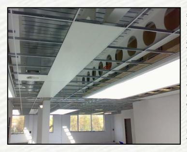
Panels are manufactured, sized for fitment within a standard 'T' bar grid. Nominal 600mm panels actually measure 594mm. These are supplied in modules of up to 3000mm. Where a longer run is required, panels are sized so that joins coincide with the ceiling 'T'. These joins are concealed with a bespoke 'H' extrusion which can be utilised in both standard and mini 'T' ceilings, having flanges of differing widths. Panels are generally fitted by
