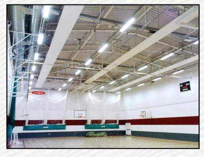
These are mainly used in sports halls but sometimes in other areas with high structural ceilings. The panels are supplied with colour matched end caps to close off the end of the panel. Joins are covered with the same extruded 'H' as the grid panels.
